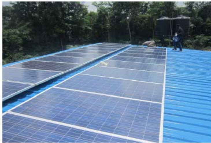
Fig 1 PV Roof Top 7.4KWp Installation
