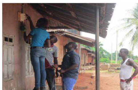
Meter installation Team
