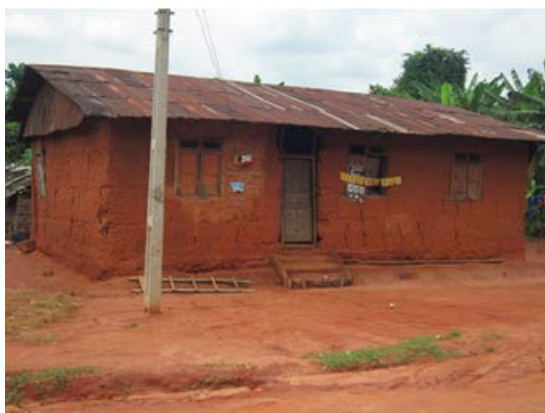
Fig 5 Circutor Dispenser meter installation
